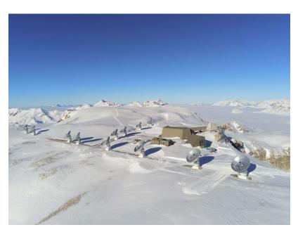
The Northern Extended Millimetre Array (NOEMA) operated by ORP Partner IRAM reached its full sensitivity with the commissioning of its 12th antenna.
